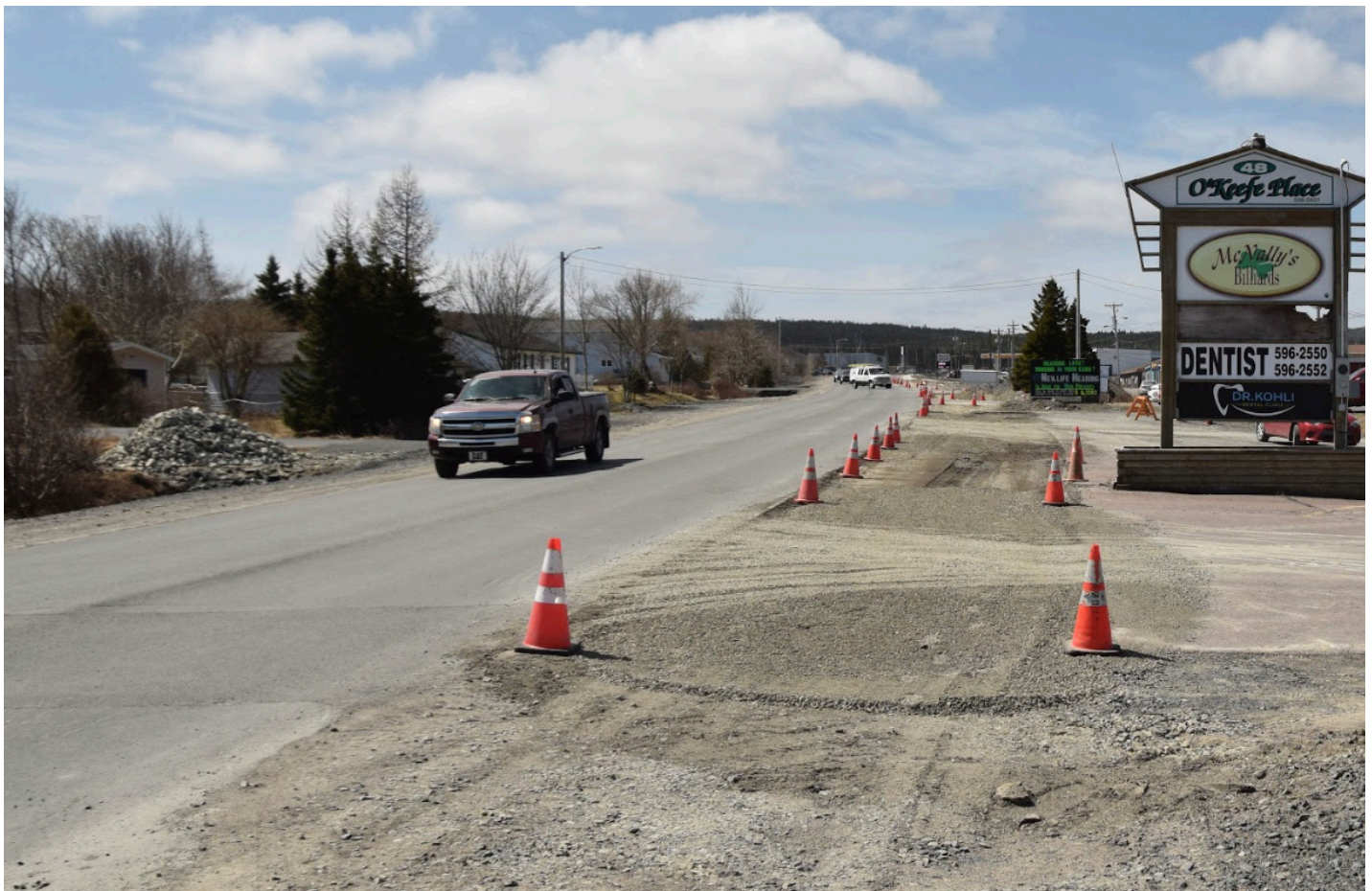
Fig 14. Sidewalk construction in Carbonear on May 2 2023.
